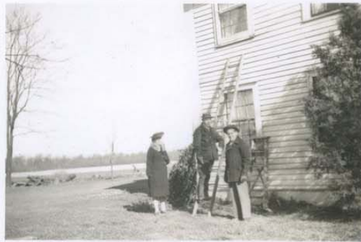
Putting up the storm sash The John Bryan Home
